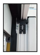
Fit the first door onto the track – DO NOT glaze at this point
